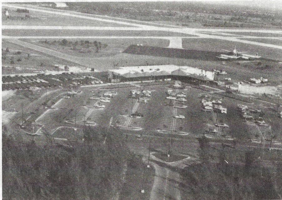
Aerial view looking north at the new Naples Airport Terminal complex. The PBA maintenance hangar may be seen at upper left.
